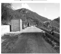
A huge project is underway in Grand Fond, with new water pipes being put in, as well as planning for underground electric and telephone wires before the new road is put in. The stone walls along the road are also being repaired or replaces and a sidewalk will be installed as well.
