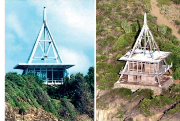
The original tipi, and its condition after Luis; Irma completed the destruction of this curious structure built by Rockefeller for his guests.
